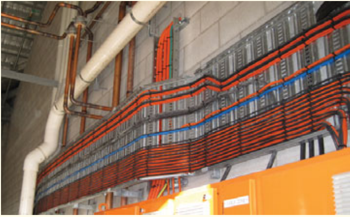
Waste Piping Can Be Routed Over-head, Horizontally
