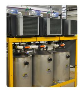
future waste loads. In all cases, the Vac Centre waste collection tanks and vacuum pumps are always selected and designed to provide redundant capacity. The Vac Centre Controls automate the operation of the vacuum pumps which run only on demand as required to restore vacuum pressure to the waste collection tanks and piping network. Optional features allow remote visibility of the system operating status as well as visibility and control of individual valve operation.
